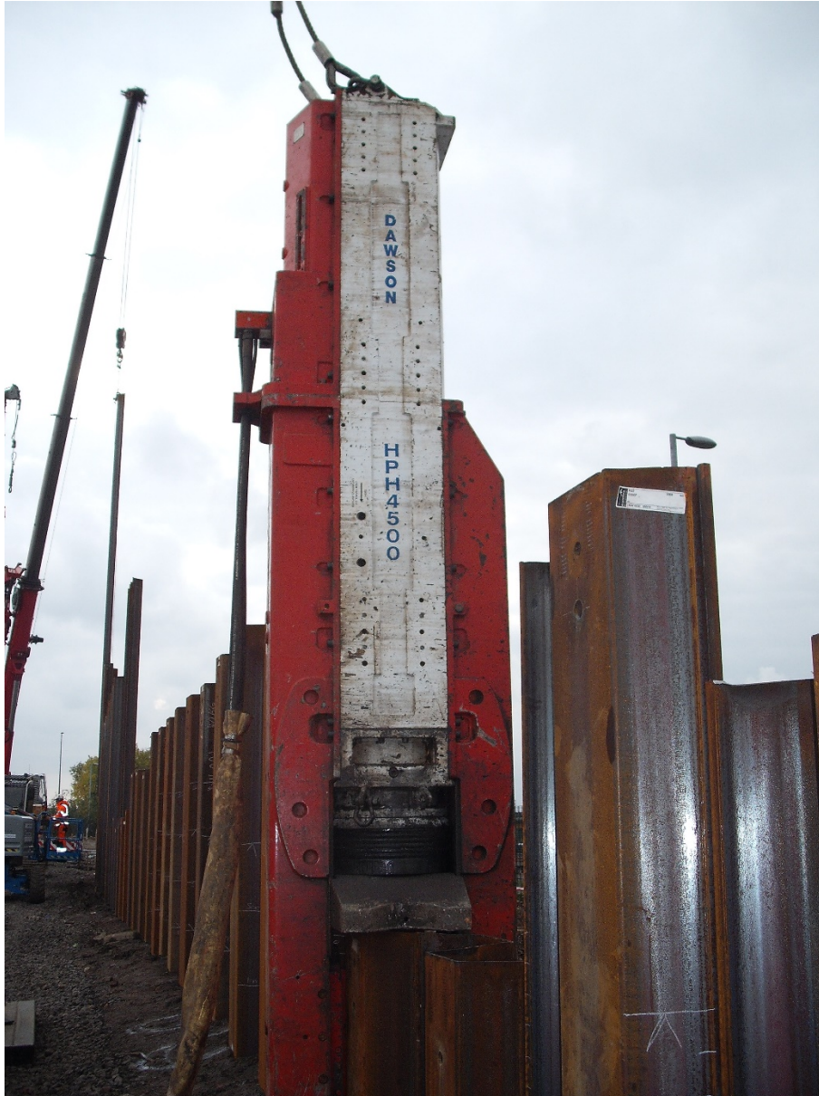
Figure 2 - Impact hammer in the field driving PU32 +1 sheet piles
