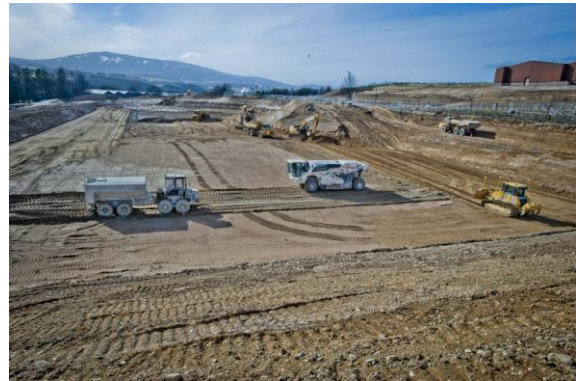
Figure 2. Specialist plant used in soil modification (courtesy of Ground Developments Ltd)
