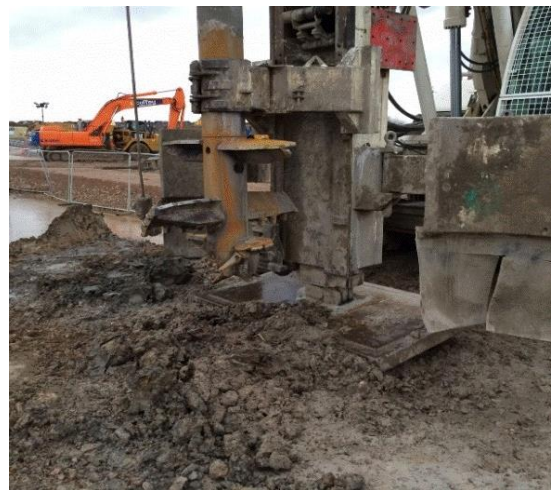
Figure 2. Turbojet mixing tool (courtesy of Ground Developments Ltd)
