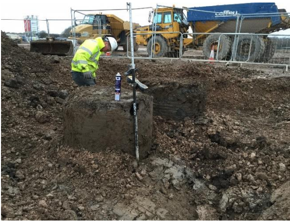
Figure 6. Exposed soil mixed column (courtesy of Ground Developments Ltd)
