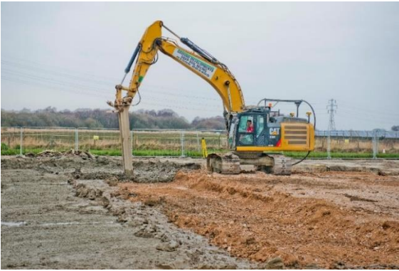
Figure 3. Mass mixing system (courtesy of Ground Developments Ltd)
